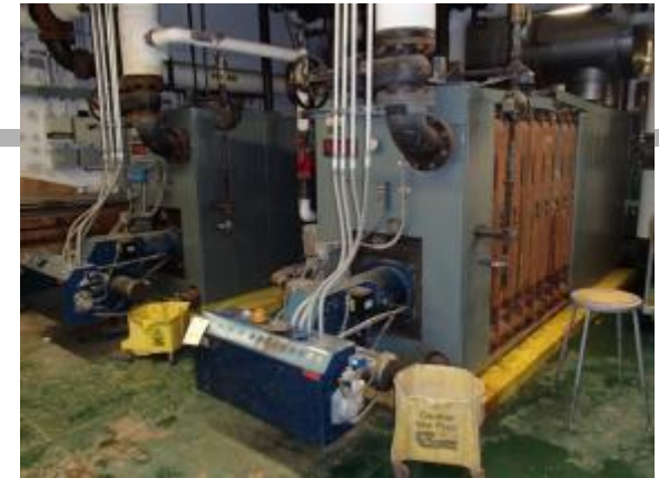
5,862 MBH Boilers in the High School
