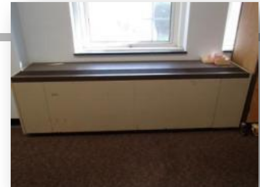
Typical Classroom Unit Ventilator
