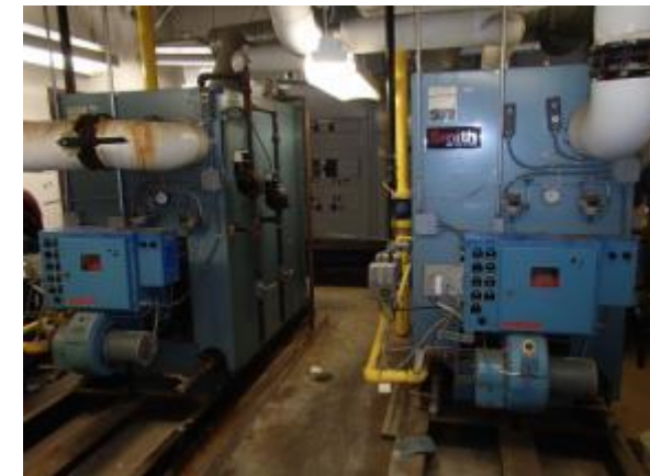
2,163 MBH Boilers in the High School
